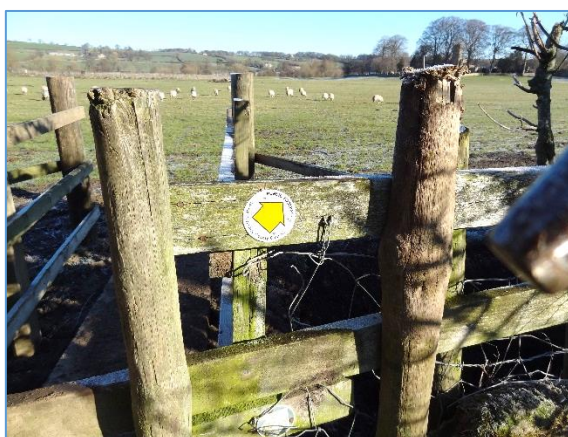
The faded waymark at bottom needs removing.
