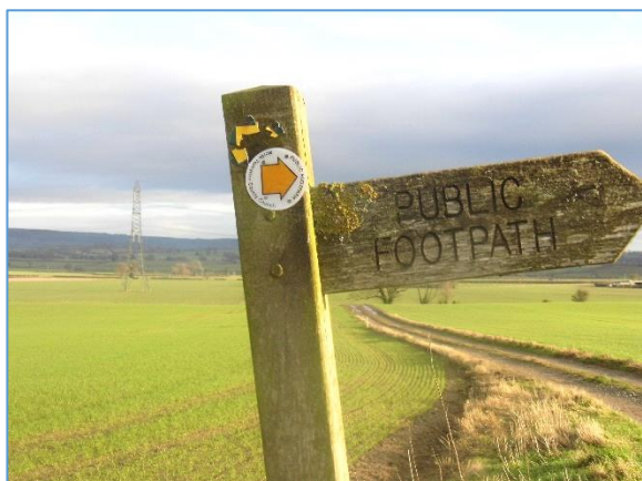
Waymark on signpost – not necessary. Old waymark has not been fully removed. New waymark is not central and overhangs the edge.
